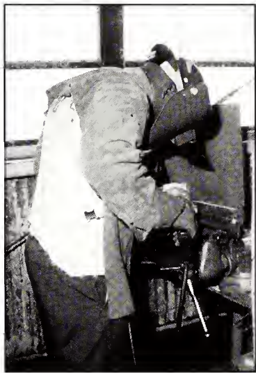
This young man welds metal posts as a part of completing a new project on fencing. (right)
