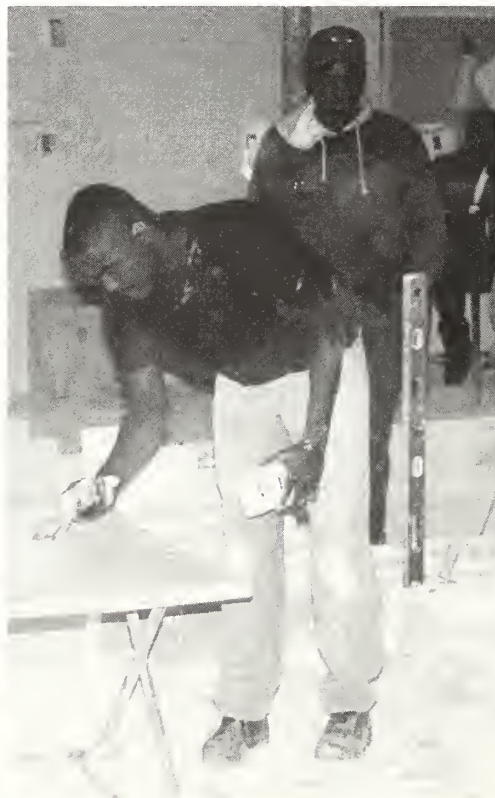
Marlon Hodges mixes the cement for the storage house foundation.
