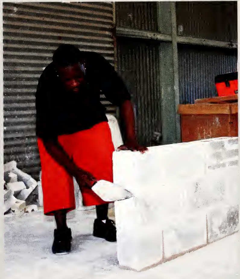
Above: Demond Noel perfects his technique by jointing his concrete blocks. Noel is also a dean's scholar.
