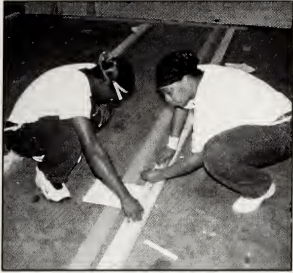
Mrs. Latosha Reed and Mr. Cardell Givens constructs a door frame.
