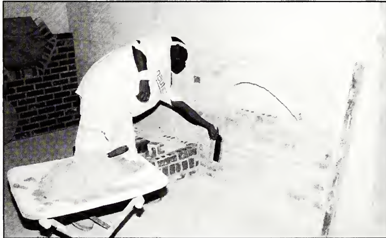
Instructor Mr. Rodney Warfield, back, shows student Derrick Hightower the proper way to cut bricks using a brick saw.
