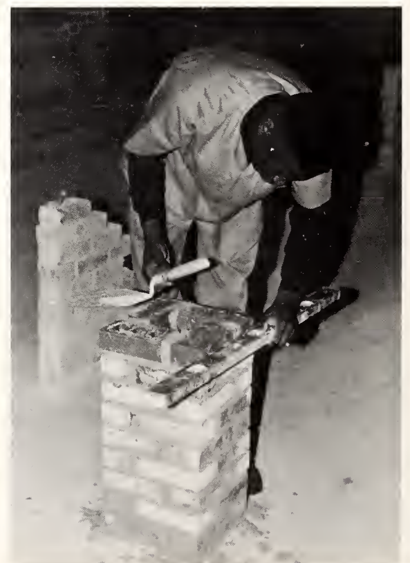
Chris Johnson puts the top layer on a practice job.
