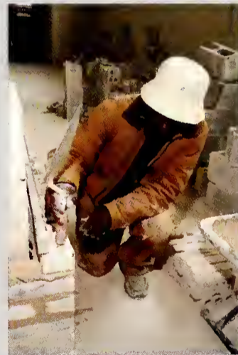
(far left) Timothy Jernigan checks wall to make sure all joints are sealed. (Left) Toni Curtis builds a corner lead as a guide for a brick wall.
