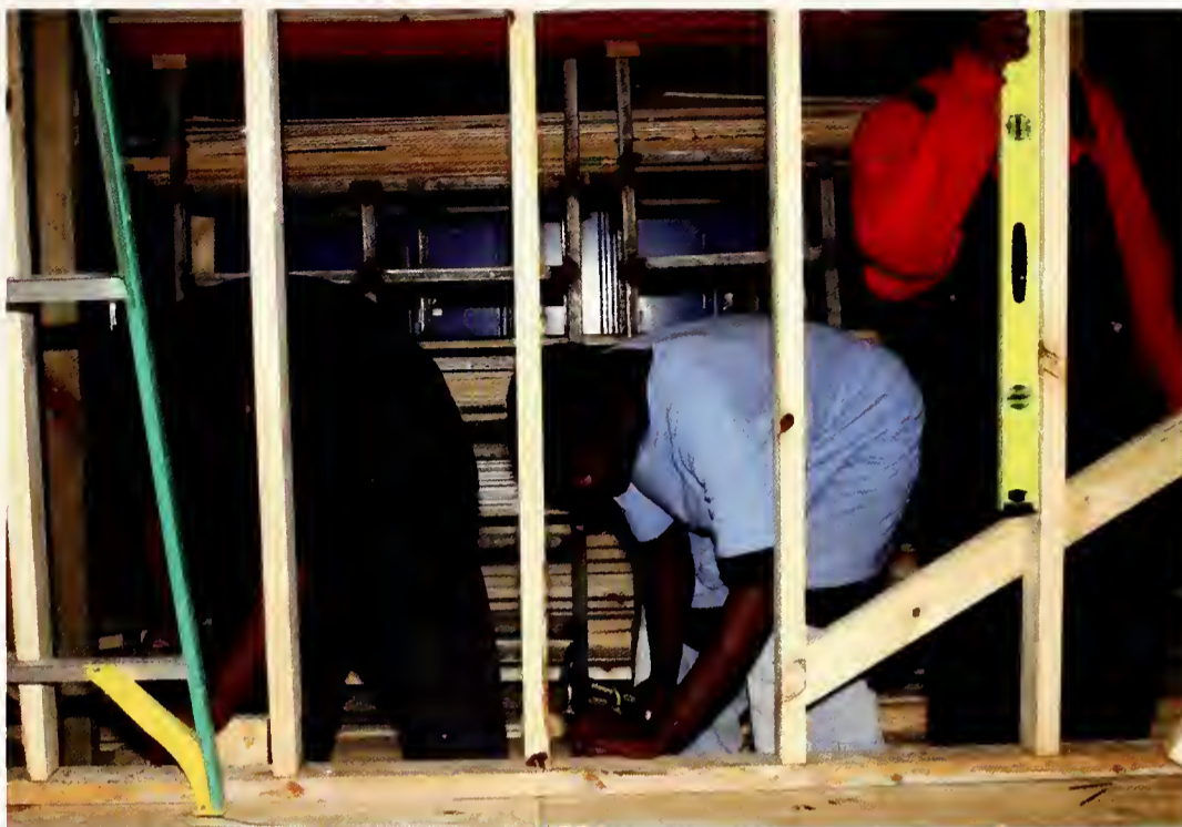
(left) LaWanda Hampton and Rolando Ward work as a team to install outside ceiling joists on a house the second-year students built.
