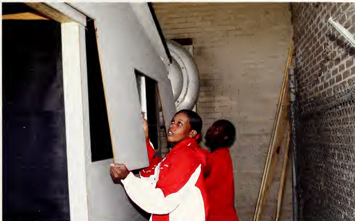
(above) LaWanda Hampton and Rolando Ward hang outside siding. (left) Henry Mosley removes a stud to install a door.
