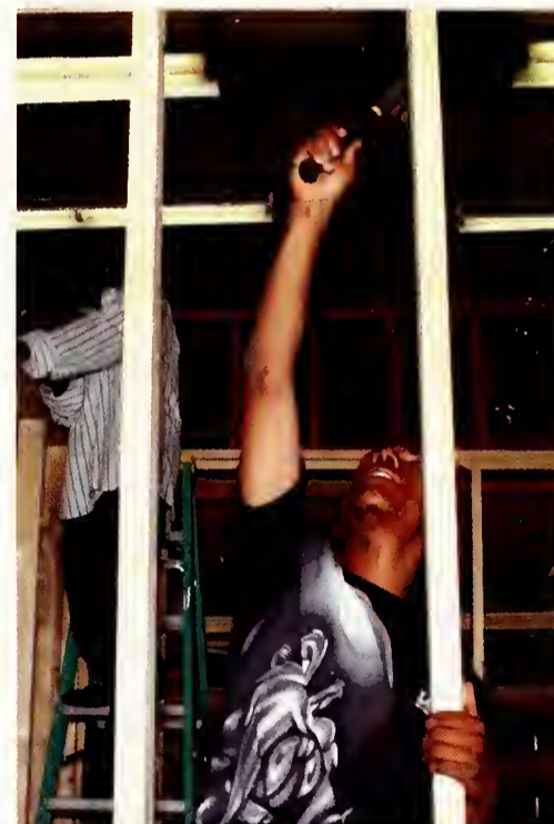
(above) As Henry Mosley carefully removes a stud, his classmates work on other areas of framing.
