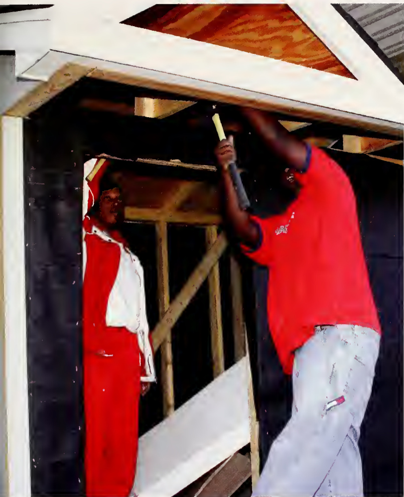
(left) LaWanda Hampton and Rolando Ward work as a team to install outside ceiling joists on a house the second-year students built.
