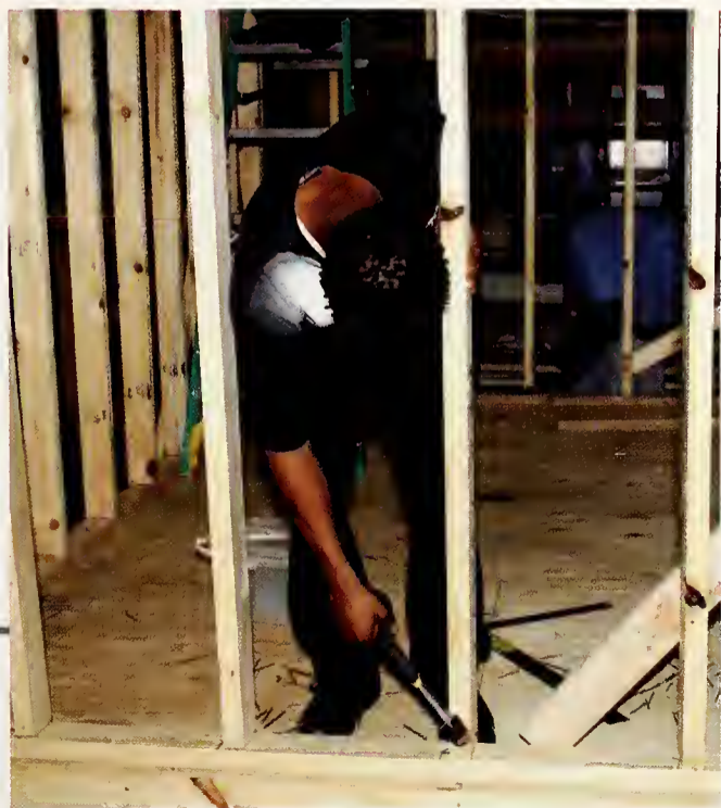
(above) LaWanda Hampton and Rolando Ward hang outside siding. (left) Henry Mosley removes a stud to install a door.
