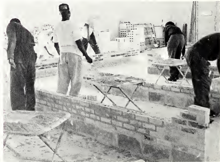
The Masonry class hard at work.
