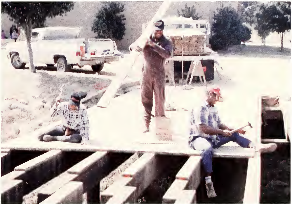
Repairing our ole faithful bridge is the maintenance crew.
