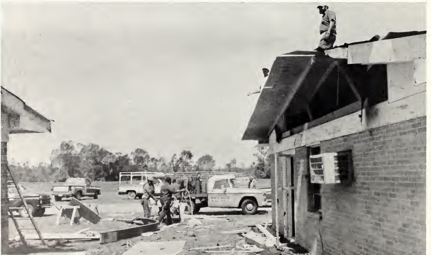
Workers repairing damage done by the tornado.
