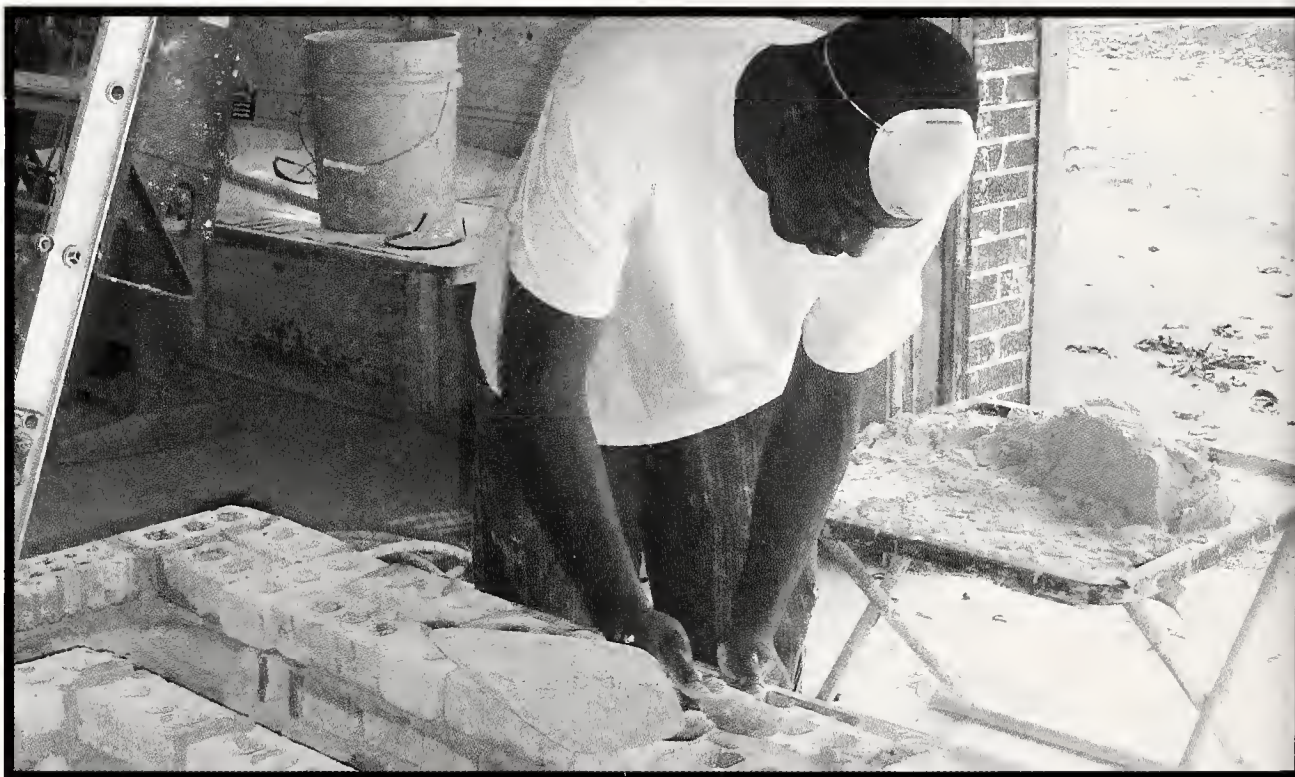
(clockwise) Ernest Marble and Marcus Roper get measurements. (right) James Tate constructs a fashionable mailbox as a class project. (above) A student aligns bricks as he perfects his brick masonry skills. The mask he wears is used to help prevent mortar dust from affecting his breathing as he works with sand and cement. The students take pride in completing the projects on which they are working.
