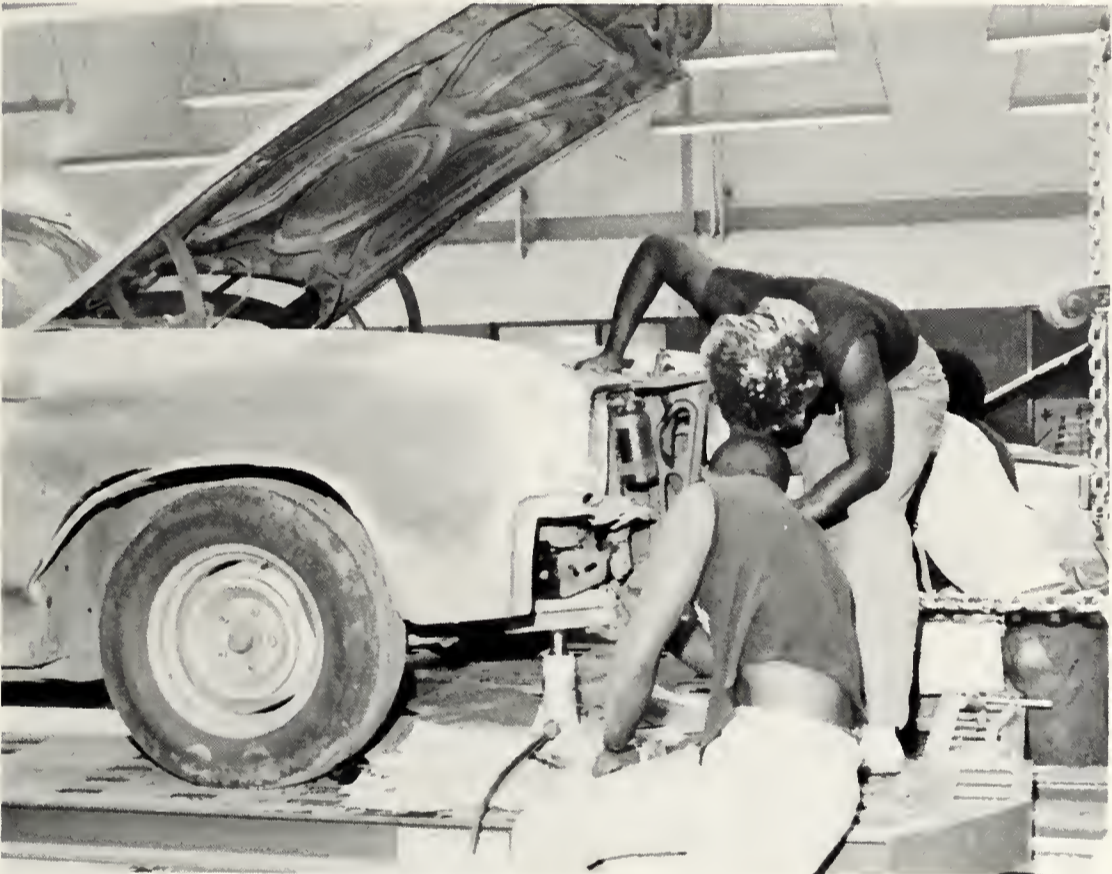
Auto mechanic student work on aligning the front end of chevrolet.
