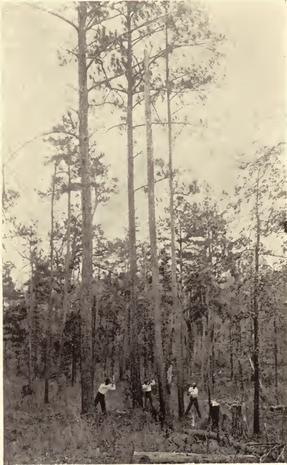
Principal Holtzclaw and the farmers felling the trees used in the construction of the first schoolhouse at Utica
