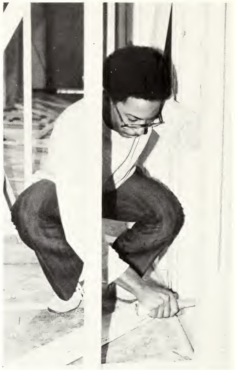
Randy works on framing a model house.
